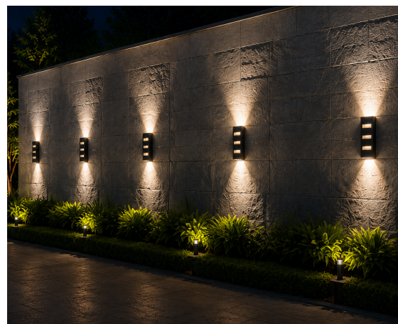
Feature Wall Lighting
